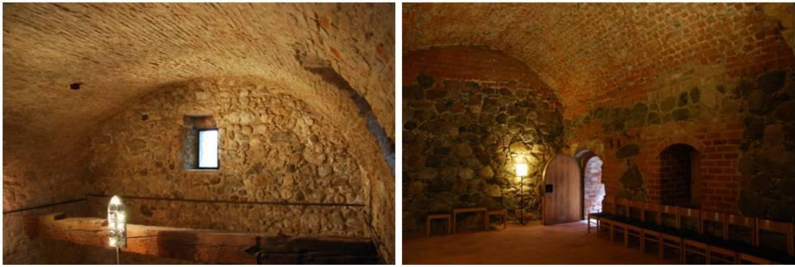
Similar barrel vaulted ceilings from the two castles. On the left from the castle of Desenzano del Garda's tower, on the right from one of the Häme castle's oldest remaining parts.
