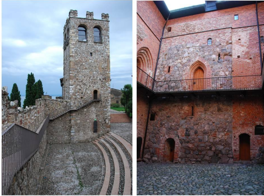
On the left, the entrance tower of the castle of Desenzano seen from the courtyard. On the right, the stone remnants of the Häme castle's entrance tower can be seen in the brick wall from the courtyard.
